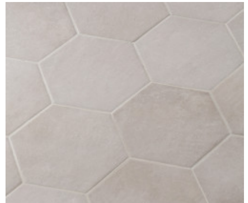
Floor grouted with Keracolor FF
