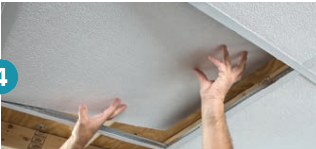
Install ceiling panels
