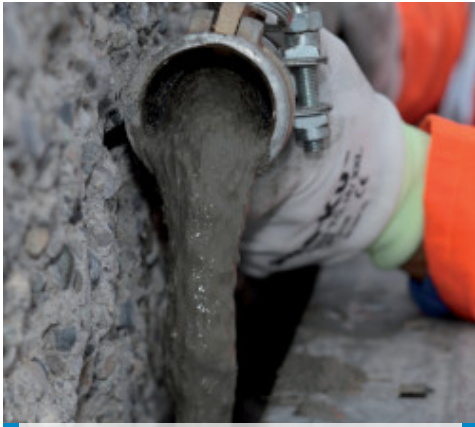
Application of Mapegrout Hi-Flow GF
