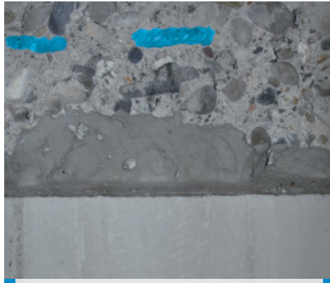
Mapegrout Hi-Flow GF after stripping the formwork
