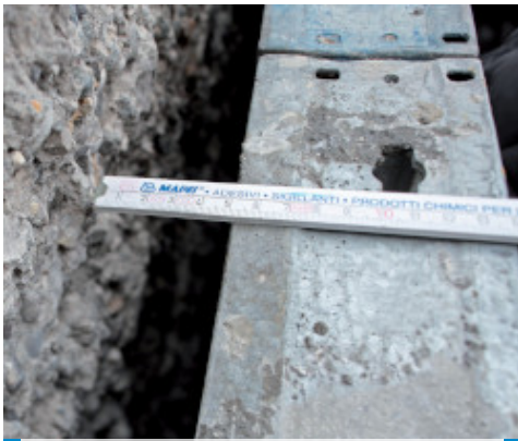
Positioning the sealed formwork once it has been carefully prepared
